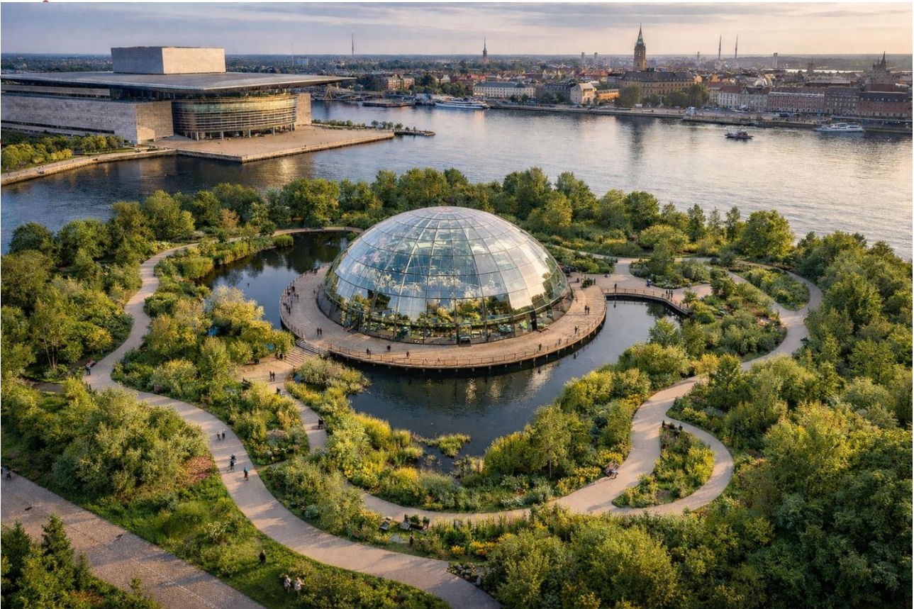
Figure 2. Ecological Integration in Copenhagen Opera Park.
